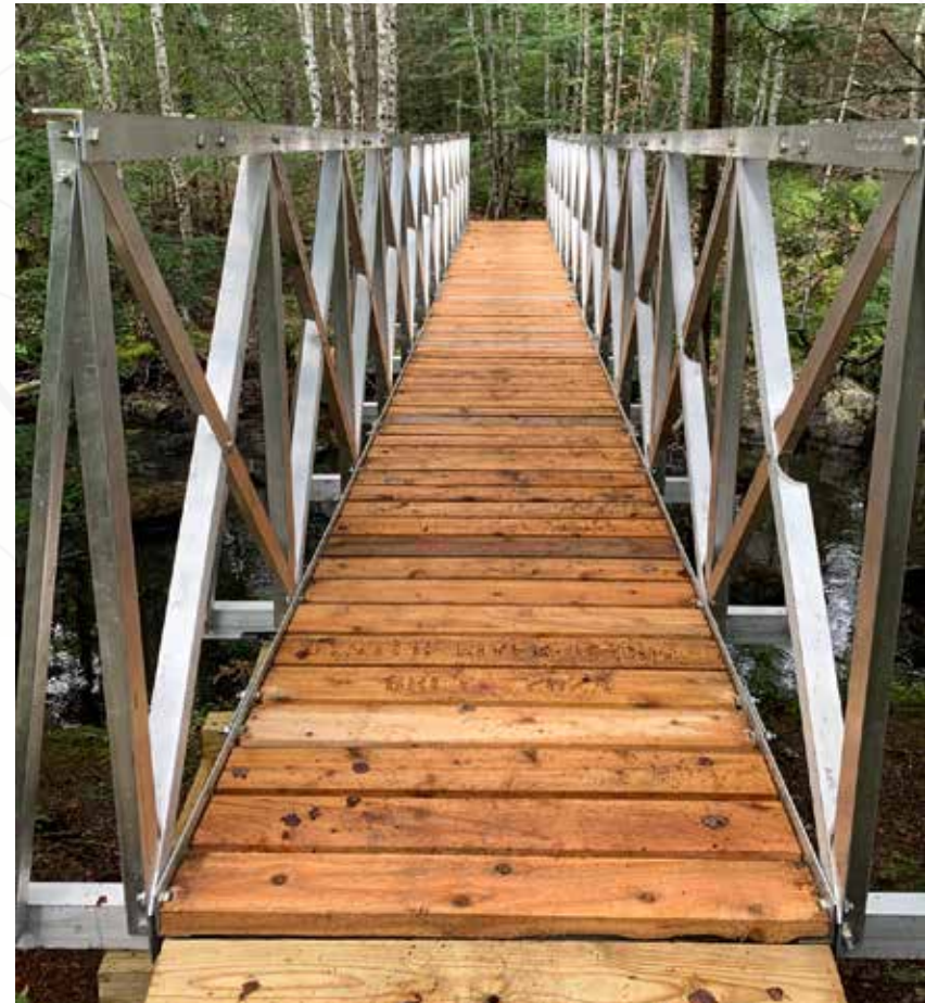
AFTER: New Bridge with restored access to a 7-mile trail
