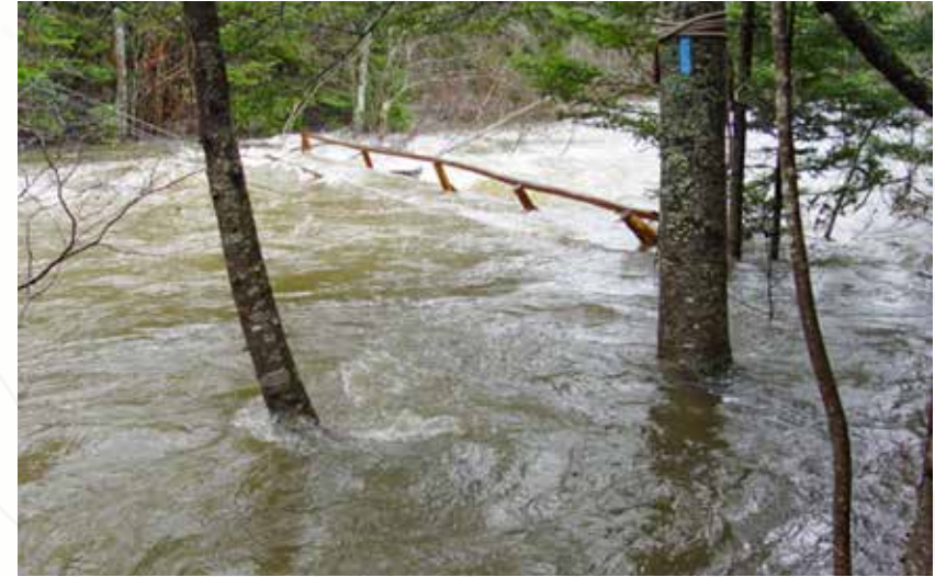
BEFORE: Washed out Oyster River Bridge
