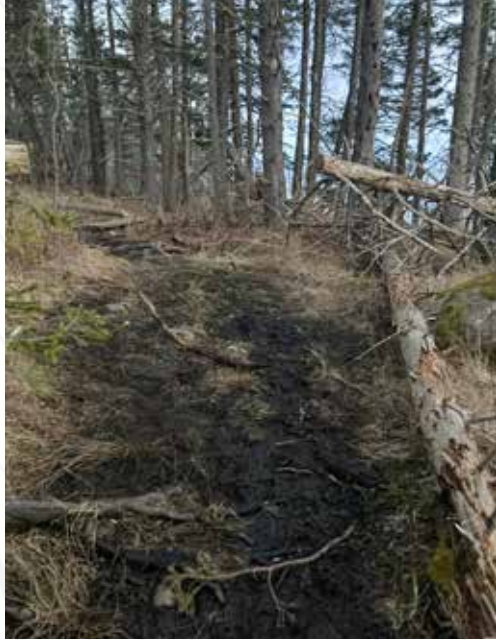
BEFORE: Wet, Widening Trail
