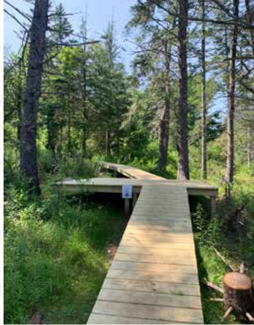
AFTER: 200 ft. of Boardwalk and Deck
